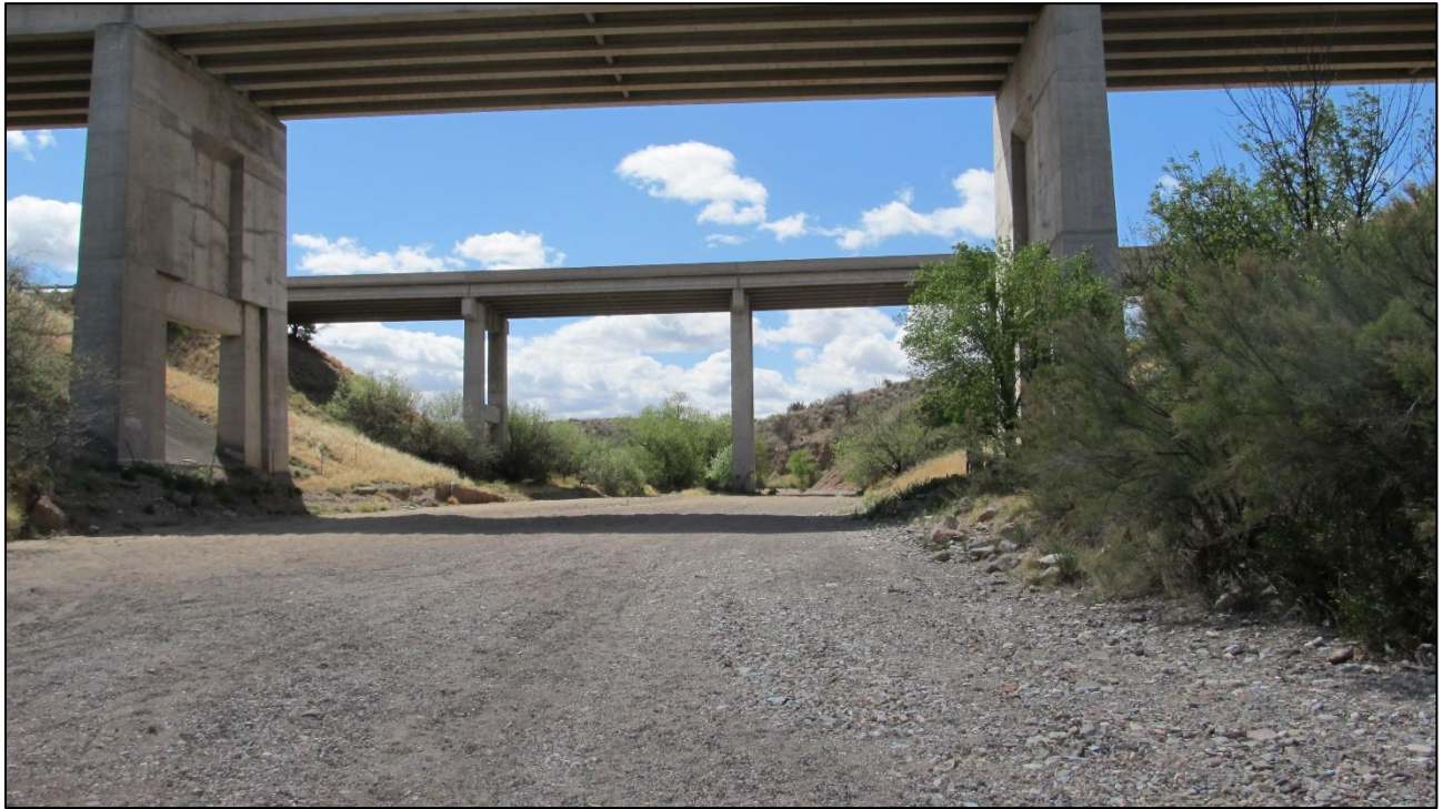
Figure 2. Davidson Canyon, east and west bound bridges, March 2017.
