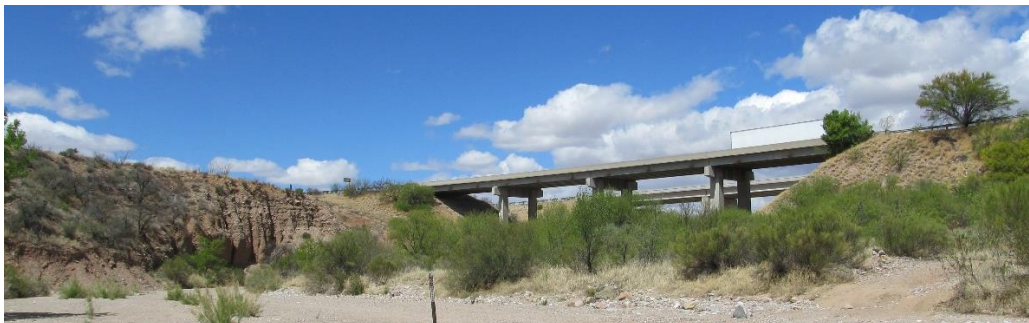
Figure 15. Looking north at the east and west bound bridges of Davidson Canyon.
