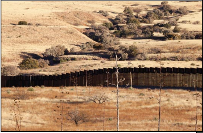
In 2009, the Department of Homeland Security replaced the vehicle barrier in Coronado National Memorial with a solid pedestrian wall, blocking passage for most terrestrial animals.
