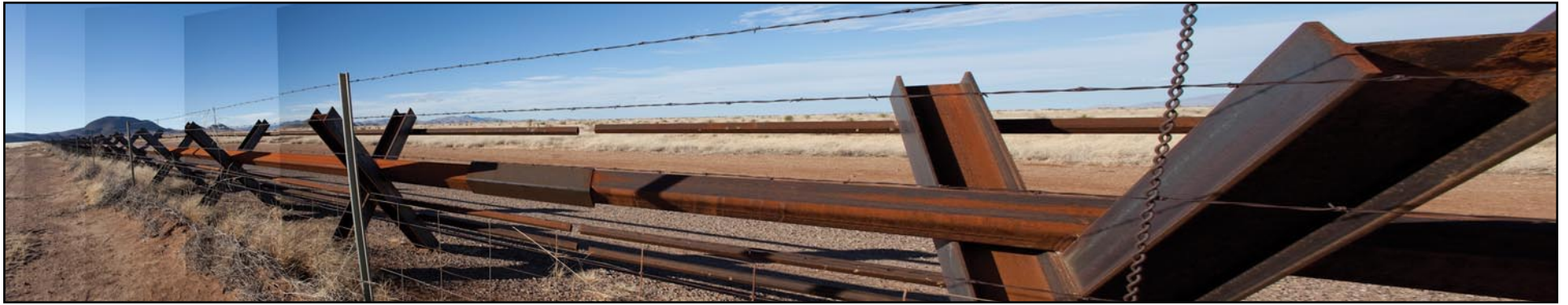
Had environmental laws not been waived, wildlife scientists could have counseled the Department of Homeland Security about minimizing obstructions for wildlife. This vehicle barrier in the Playas Valley of New Mexico/Chihuahua could have been built in a manner that afforded passage to wildlife like bison, pronghorn and deer. But without input from the wildlife conservation community and the public at-large, the border barrier now blocks passage by most large mammals.
