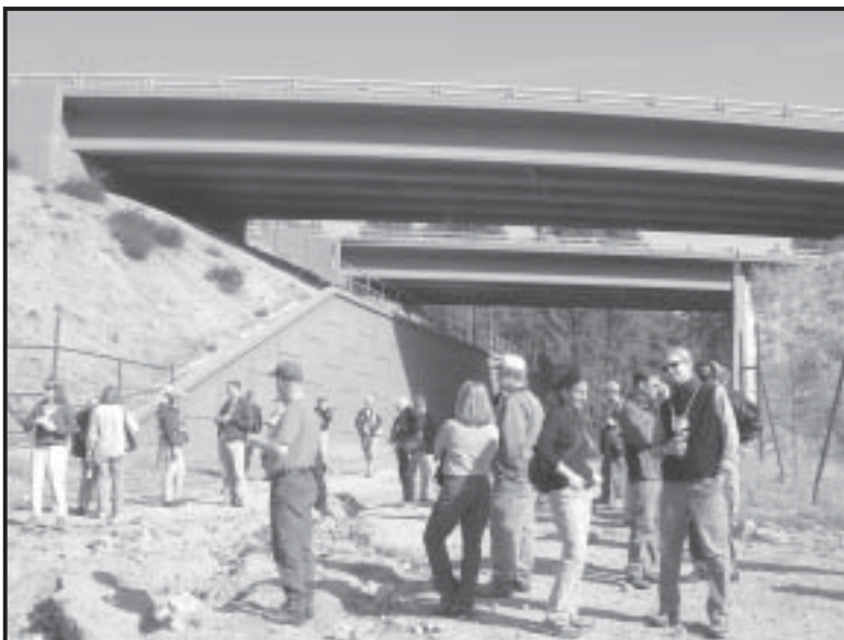
Researchers speculate that this type of culvert inhibits elk from passing by providing a ledge upon which predators may hide.
